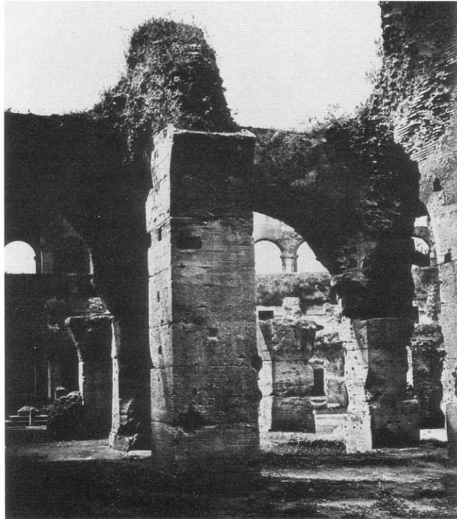
Figure 16 Robert Macpherson. Broken Arches in the Colosseum , before 1860. Albumen print. Collection Phyllis Lambert, on loan to the Canadian Centre for Architecture, Montreal.
